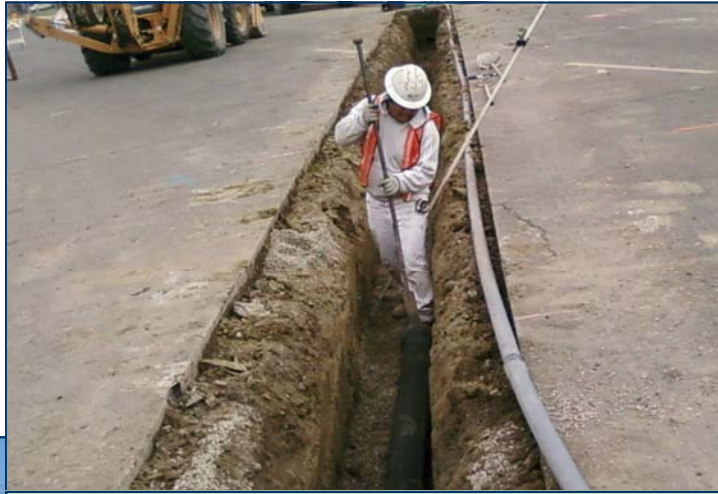
NEWMAN SEWER REPLACEMENT
