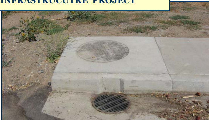
WATERFORD SKYLINE INFRASTRUCTURE PROJECT
