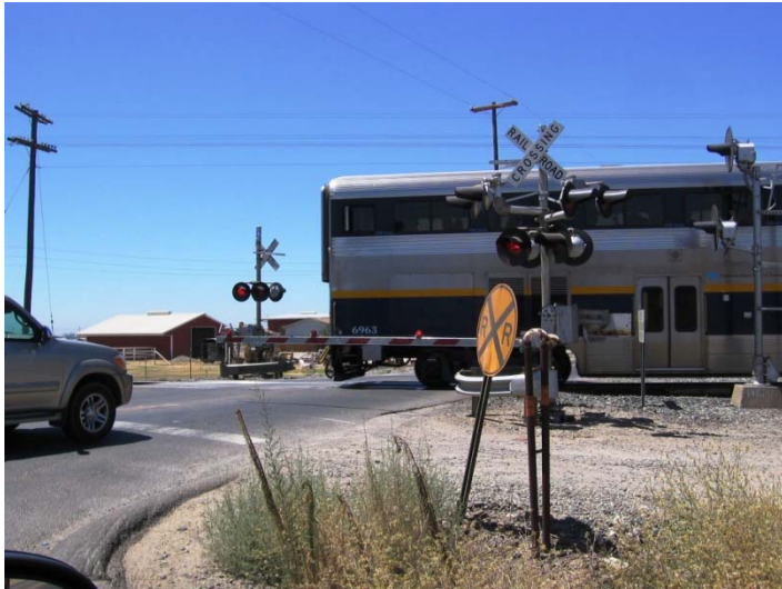
Unsafe railroad crossing; no curb, gutter, or sidewalk; overhead utility lines; weeds
