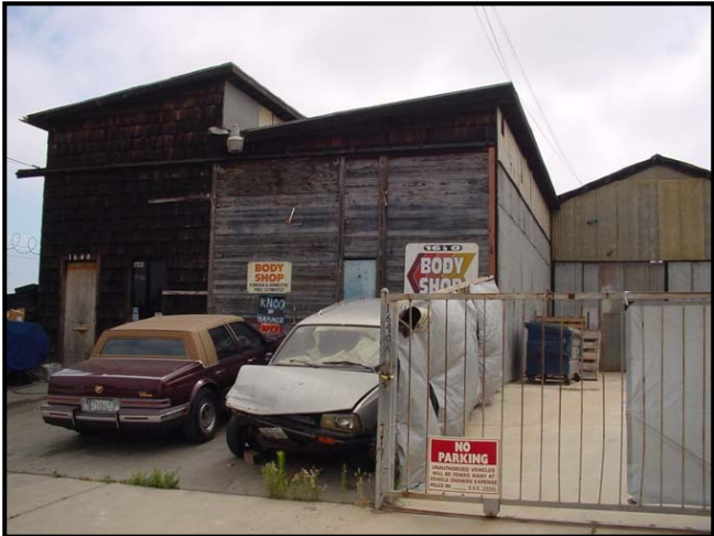
FH – Fire Hazard
