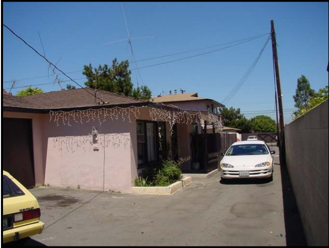
IE – Poor Site Ingress/Egress (including emergency vehicle access)
