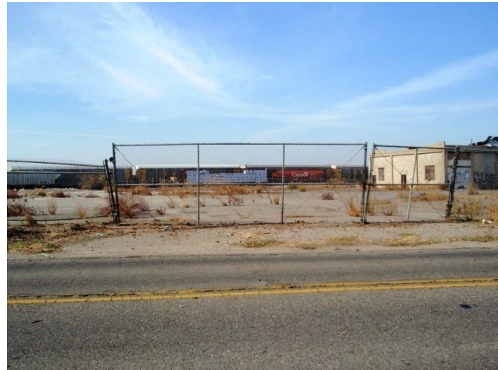
Previously developed, now vacant; damaged chain link fence; weeds
