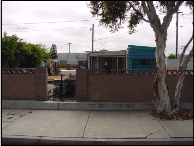
ANPA – Addition Not Permitted (Room Addition/Alteration, etc.)
