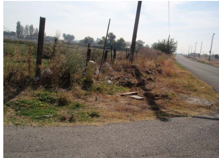
No curb, gutter, or sidewalk; damaged fence; overhead utility lines
