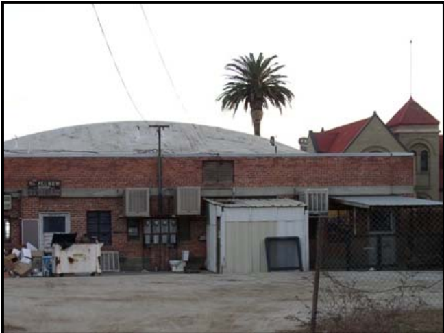
AS – Appurtenant Structure
