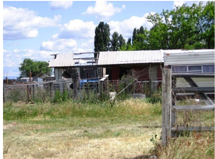
Seriously damaged and deteriorated building
