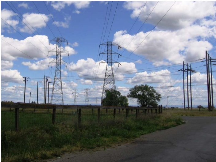
Excessive overhead utility lines; no curb, gutter, and sidewalk
