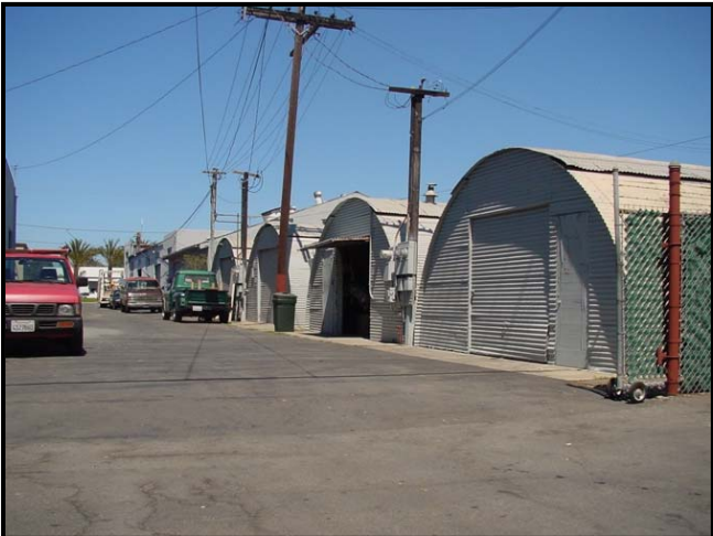
SD – Substandard Design (structure)
