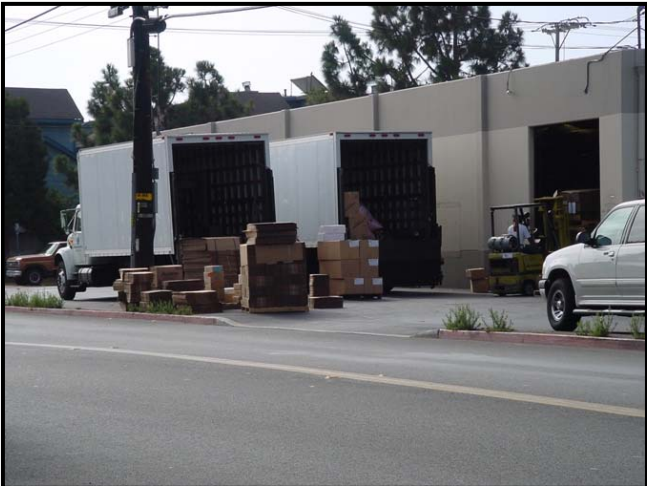
ILD – Inadequate Loading/Docking Facilities
