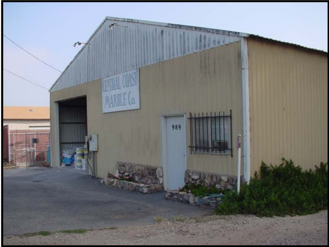
PQ – Poor Construction Quality/Corrugated Steel/Building Type
