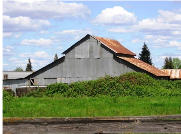
Seriously rusted building
