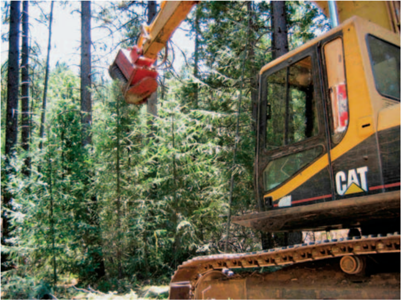
Masticators and other harvesting equipment use tree limbs to create a “slash mat” to walk on, which can protect the ground and enrich soils.
