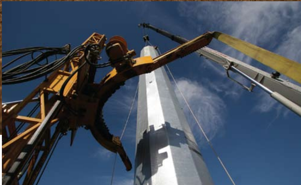
Steel towers are set as construction begins on the new Westley-Rosemore 230 kV transmission line.
