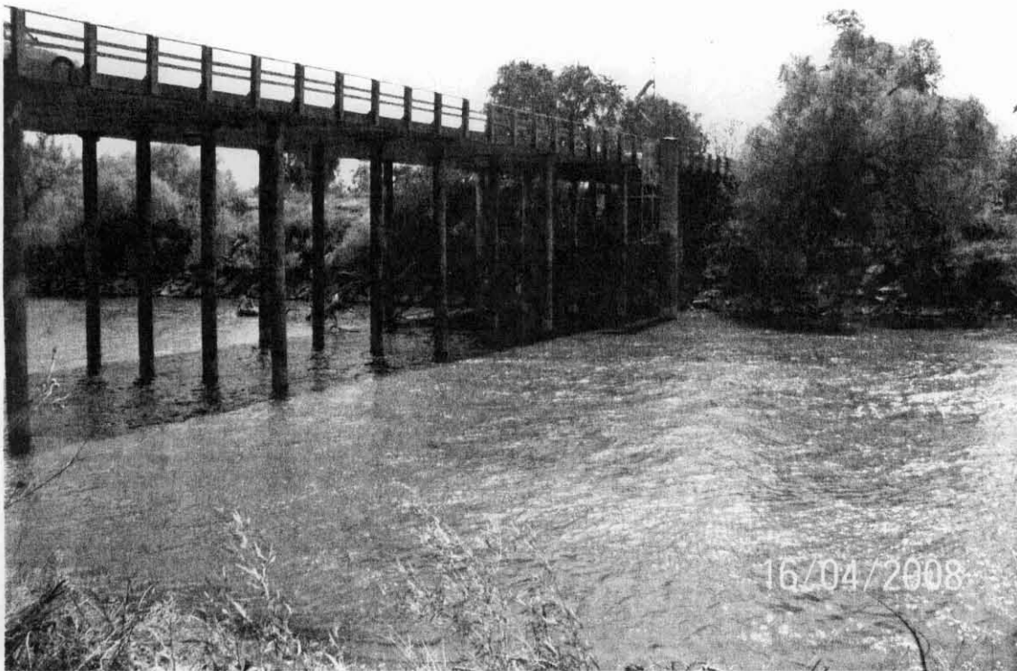
Las Palmas Road Bridge crossing the San Joaquin River; looking southwest
