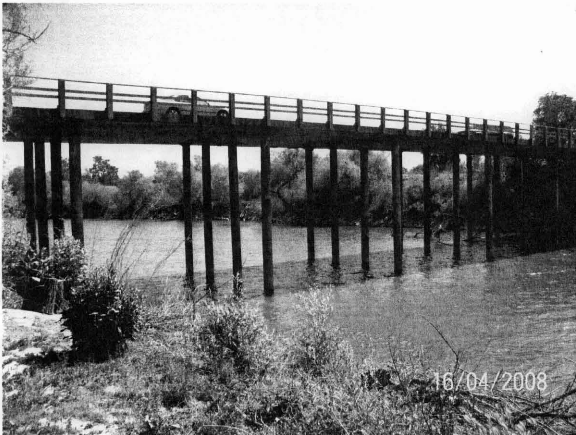
Las Palmas Road Bridge crossing the San Joaquin River; looking southwest
