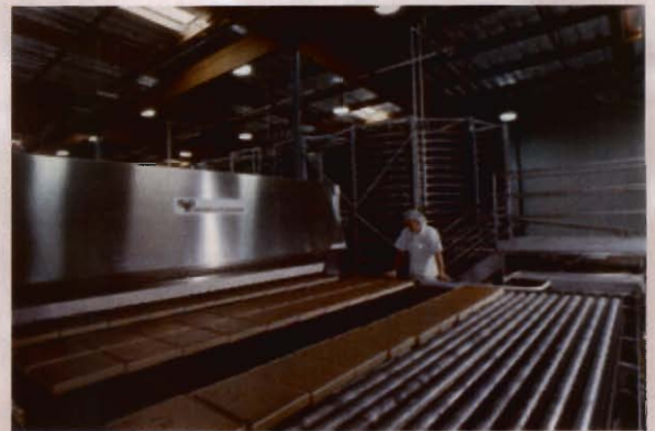
Bunge Foods Cake Processing Plant
